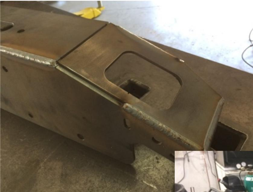
Step 5: Weld all seams, bouncing around to balance heat input as described. Once welded, you can choose to leave the welds exposed or grind them back to a nice bevel for a smooth appearance depending on your desired outcome.
